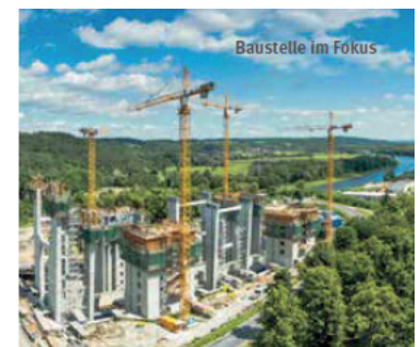
Assembly of reinforced concrete structures
